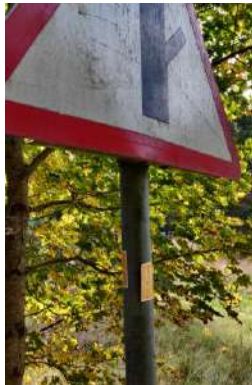
Figure 29. The sticker on the road sign post is not sticking.
