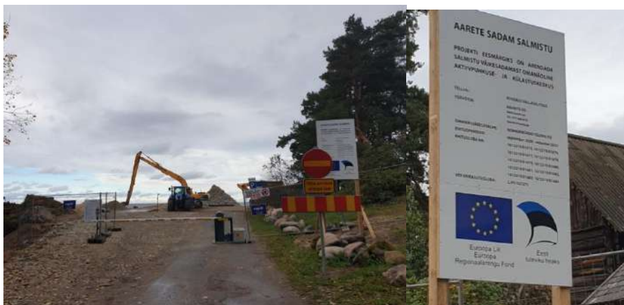
Figure 37. The construction works at Salmistu Harbour.
